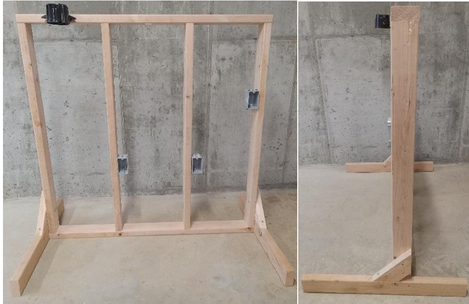
Figure 3. Framed Wall with Junction Boxes
