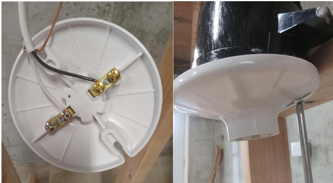
Figure 8. Install the light fixture
