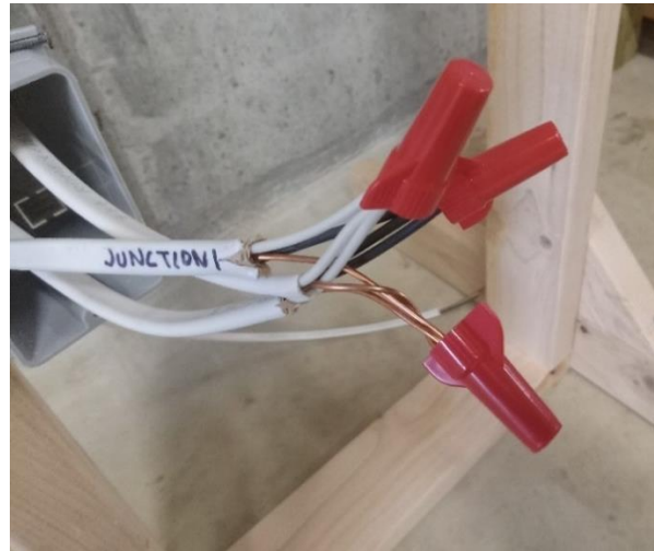
Figure 11. Connect the wires in the junction box
