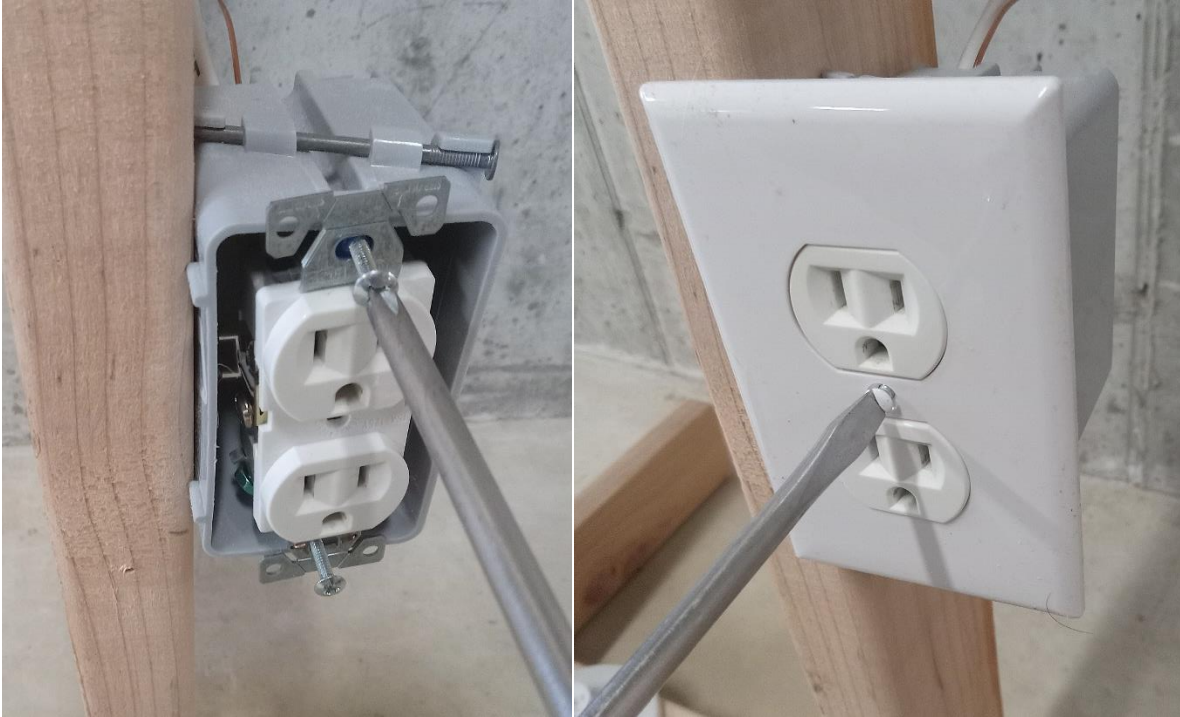
Figure 7. Secure the outlet and cover plate
