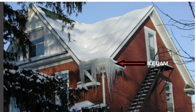
FIGURE 1. Example of an Ice Dam
