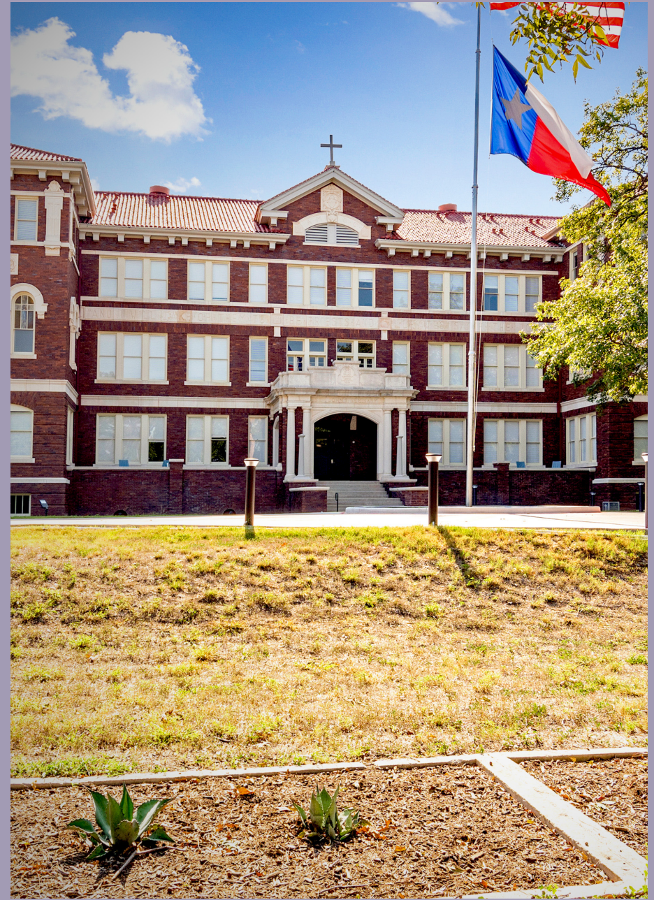
The adaptive use of the former St. John's Seminary in San Antonio, Texas, created 228 apartment homes for a range of income levels. (Paige Shinn Photography)
