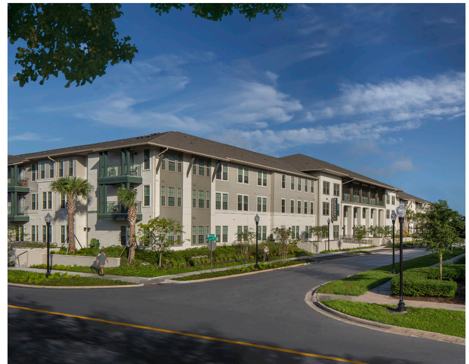
Pendana at West Lakes is the rehabilitation of hundreds of vacant and dilapidated apartments into a mixed-use, mixed-income community with 320 apartments near downtown Orlando, Florida. (Rion Rizxo/Creative Sources)
