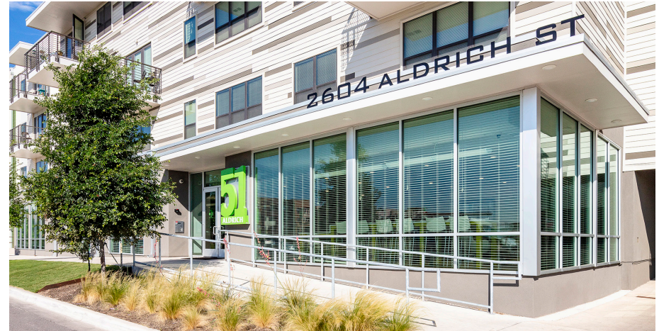
Aldrich 51 is a mixed-income workforce housing development in Austin, Texas, located in Mueller, a 700-acre mixed-use redevelopment community. (Jake Holt/Patrick Wong)
